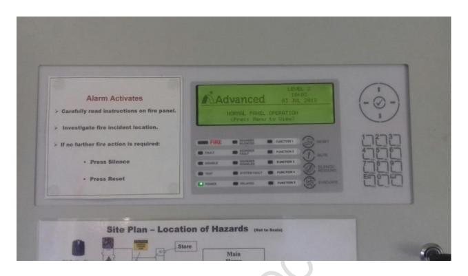
On activation, the alarm sounder will ring until manually re-set by pressing the "Silence Resound" button on the MCP. A 'Zone Plan' on the wall alongside the MCP gives easy reference to the location which correspond to the information shown on the MCP WHICH IS ACCESSED BY PRESSING right Arrow button to scroll through line by line. By pressing the silence resound button, this does not reset the system; the re-set button will do this as shown on the MCP.
