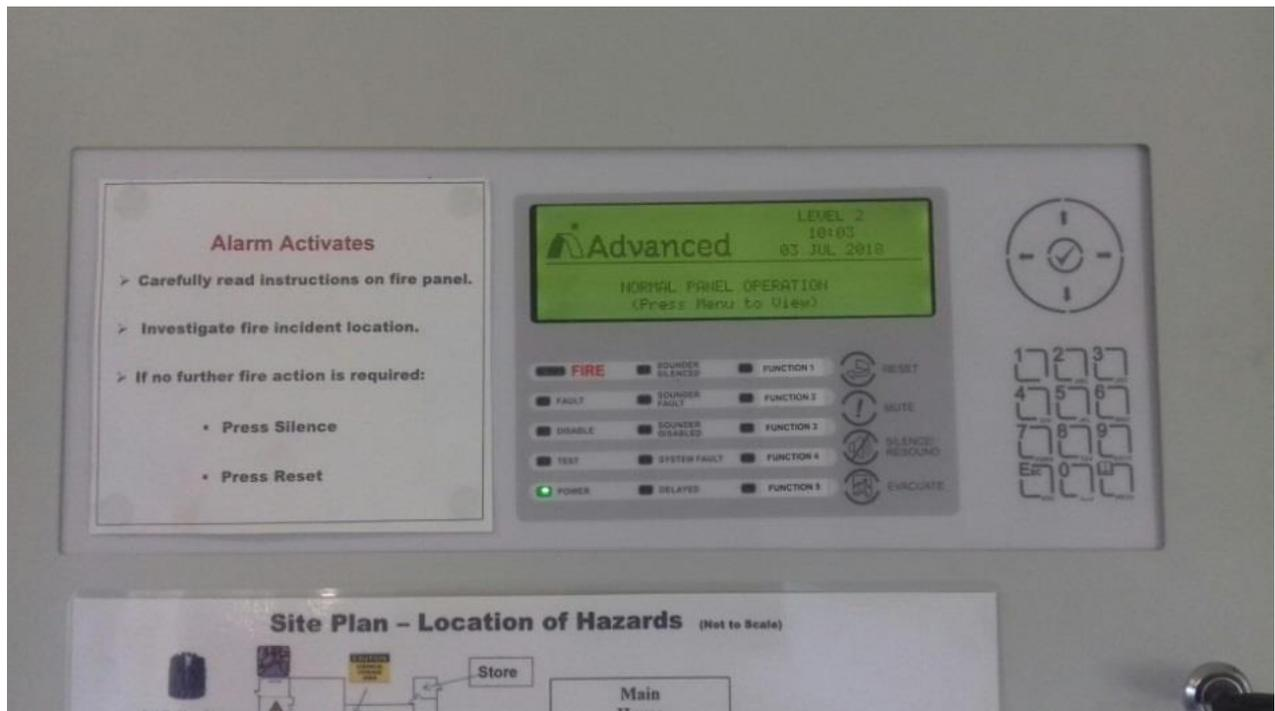
On activation, the alarm sounder will ring until manually re-set by pressing the “Silence Resound” button on the MCP. A ‘Zone Plan’ on the wall alongside the MCP gives easy reference to the location which correspond to the information shown on the MCP WHICH IS ACCESSED BY PRESSING right Arrow button to scroll through line by line. By pressing the silence resound button, this does not reset the system; the re-set button will do this as shown on the MCP.
